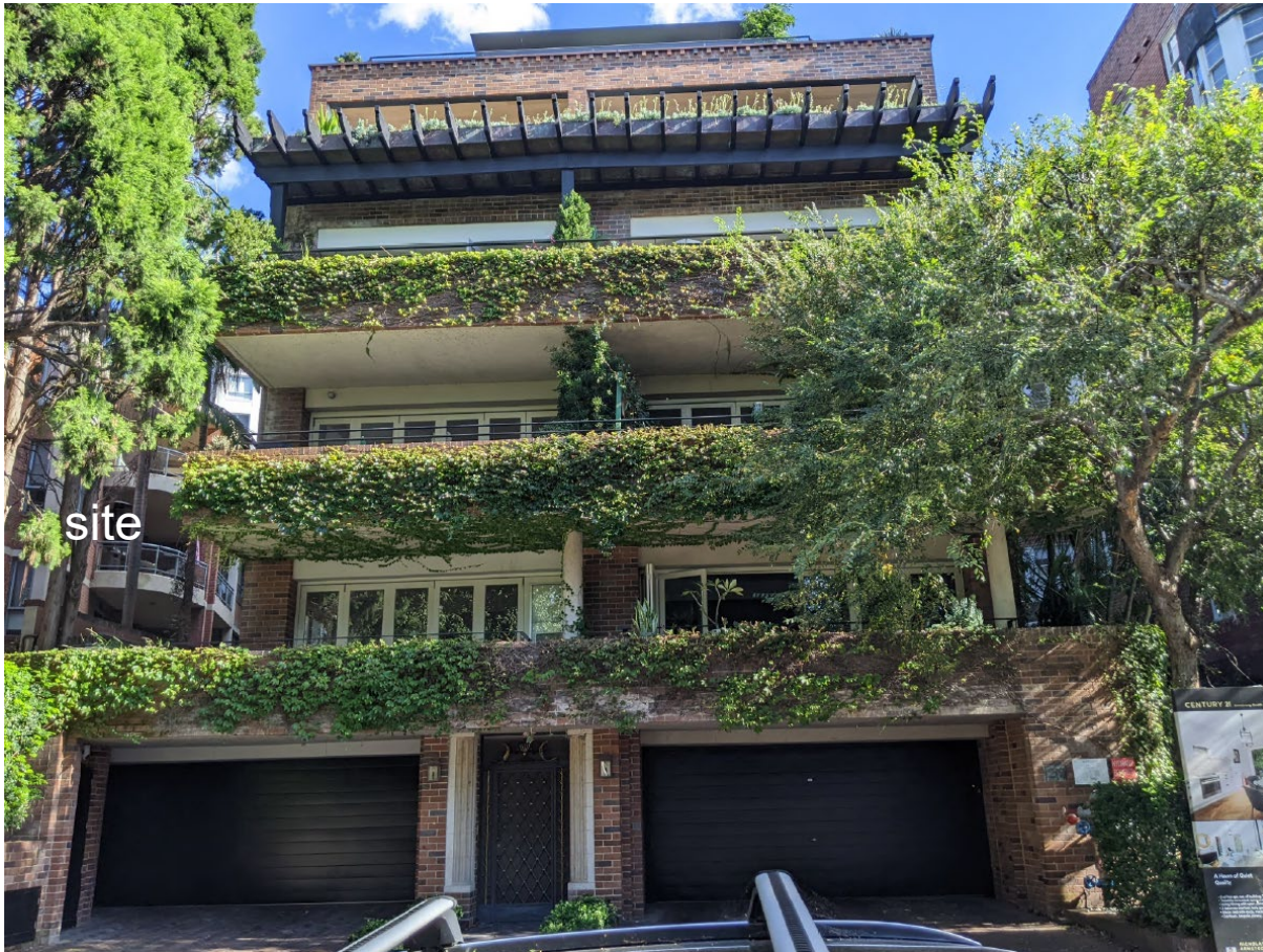
front of No.27 Billyard Avenue, adjacent neighbour to the west of the subject site
