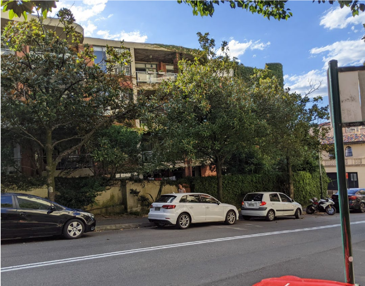
side (east) elevation of site viewed from Ithaca Road
