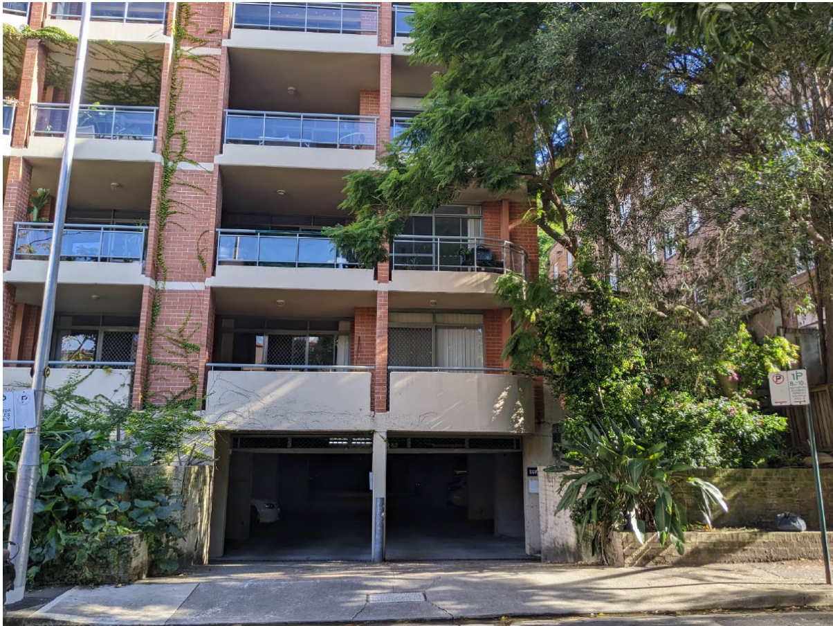
existing double crossover vehicle access to basement from Billyard Avenue
